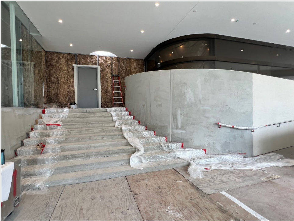
View of newly poured stairs and plaster refinishing in progress
