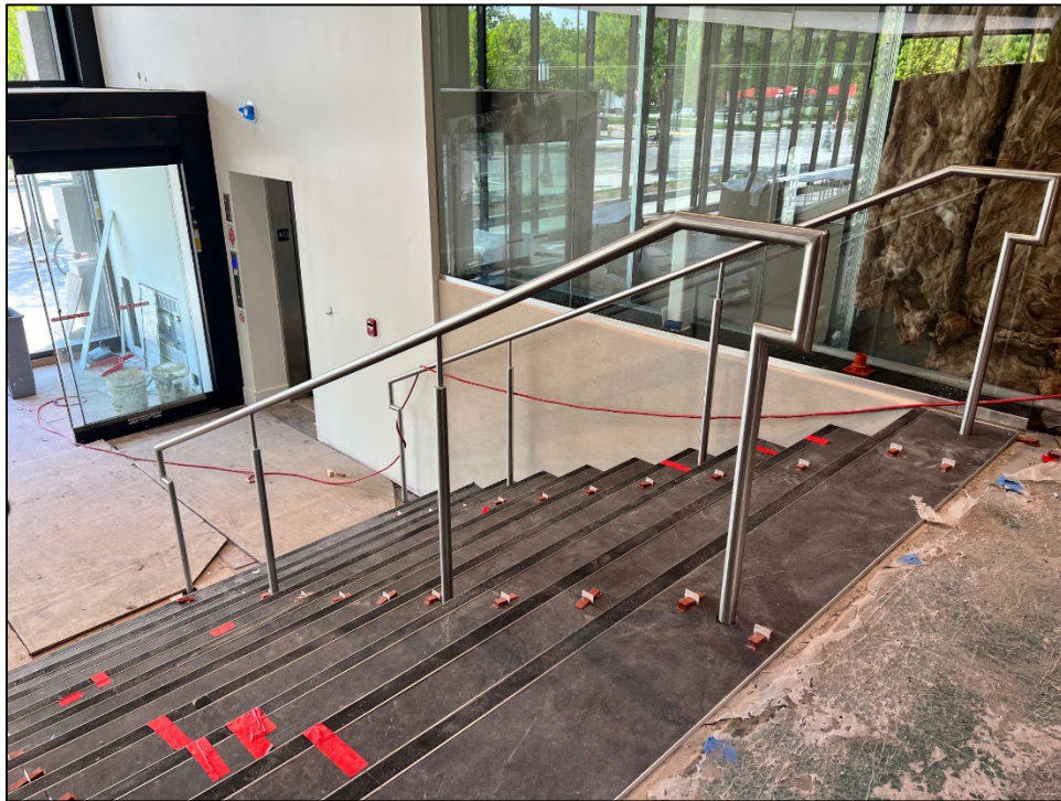
View of steps from top of ramp
