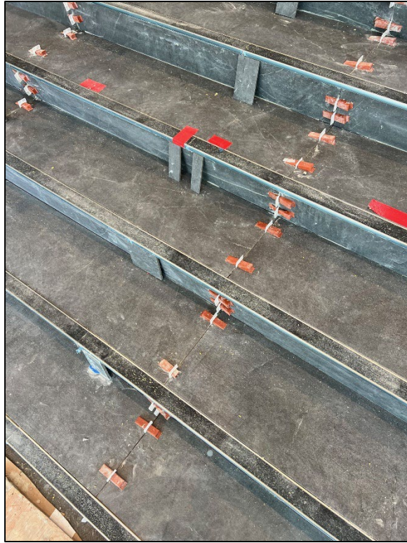
View of stair treads
