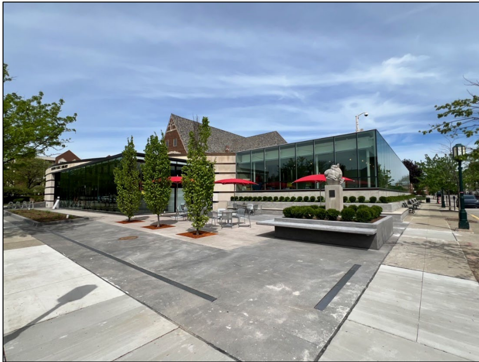
View of plaza from corner of Bates and Merrill Streets
